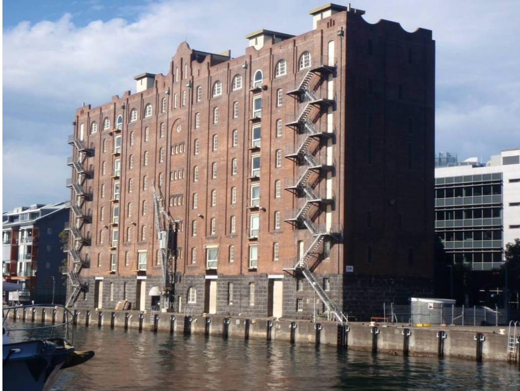
Figure 18: Existing view of Building C
