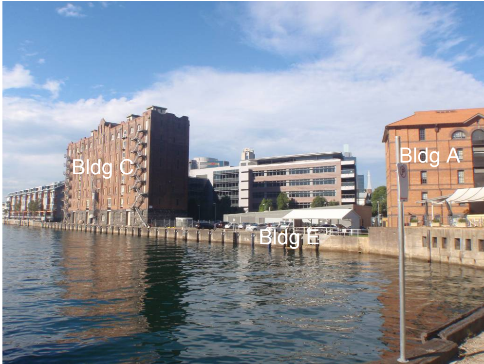
Figure 3: View of existing Building C, Building E and Building A (L to R)
