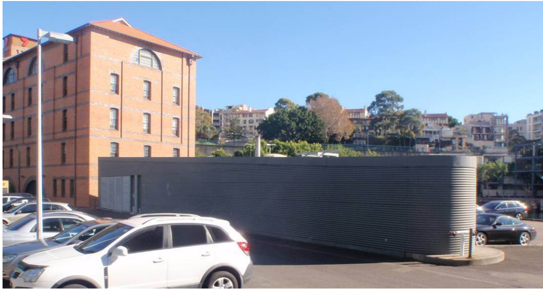
Figure 5: View of existing Building E and car parking area proposed for demolition
